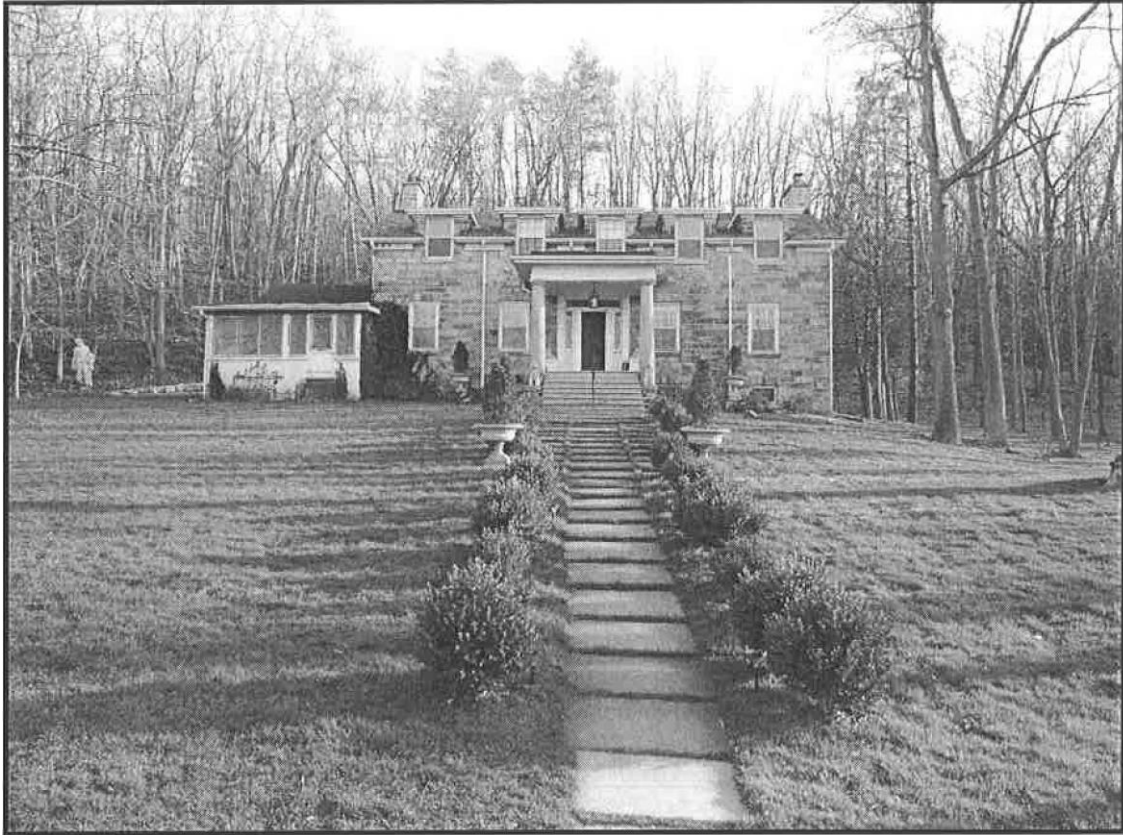
Figure 4. The above image depicts the front elevation of the dwelling at 95 Cline Mountain Road. The Georgian proportions of the dwelling can be seen by the five bay facade with a central entry and the symmetrical chimneys. The entrance is also indicative of the Georgian style with pilasters, sidelights and a shallow transom. The walkway and stairs leading to the entrance strongly define the main entryway. The portico displays Greek revival influences with the fluted Doric columns which contribute to the dwelling's distinctive character. Originally a single storey dwelling, the five dormer windows would have been added during the 1830 additions. The addition on the west side of the dwelling is not part of the proposed designation. (Source: Town of Grimsby, April 2012).
