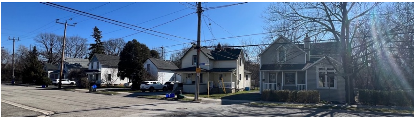
Figure 3: contextual view looking east from John Street, across Robinson Street N
