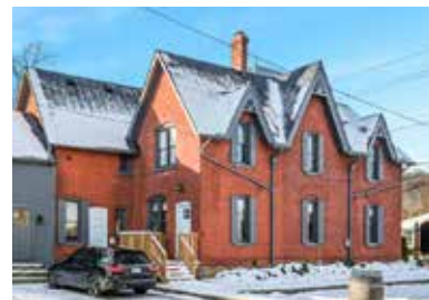
The steep gables and elongated windows of the house display its Gothic Revival style (photo courtesy of the property owner).
