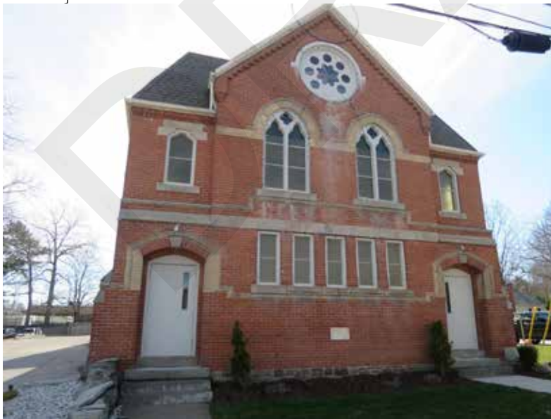
West elevation showing some masonry staining/soiling (ERA, 2021).
