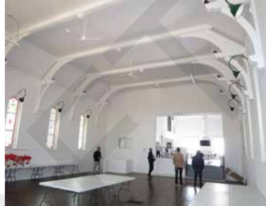
Present (2021) view from within the sanctuary space towards the 1913 Sunday School addition with raised first floor level (ERA, 2021).
