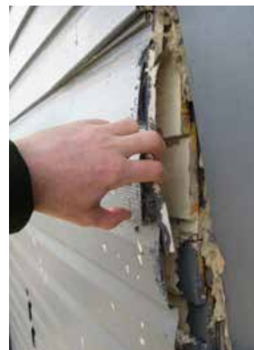
Opening in vinyl siding at rear addition/north elevation revealing wood clapboard siding beneath (ERA, 2021).
