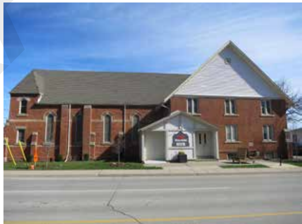
Current photo of the Church showing the south elevation of the 1880 Church (left), a later doorway addition (centre) and the 1913 Sunday School addition (right). The footprint and cross gable of the Sunday School addition somewhat obscures the original 1880 building footprint. The raised basement and first floor stand in contrast to the 1880 church building, whose first floor level sits much closer to grade (ERA, 2021).
